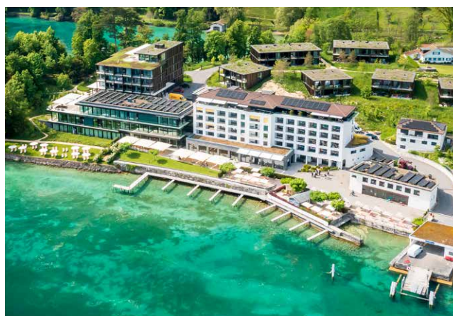
PV-Anlage Campus Hotel Hertenstein
